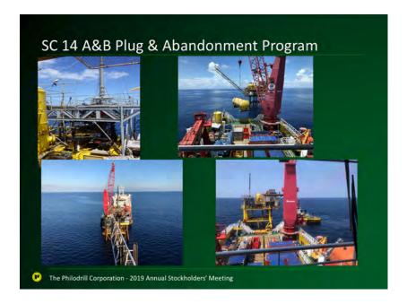
The P&A of the 9 remaining wells in Nido and Matinloc was undertaken from April to May this year. The program was completed under budget at about US\$4.7MM. However, in the Nido A1 and A2 wells, only the primary plugs across the reservoir were cemented. This required a return by early next year to complete the intermediate and shallow cement plugs on these wells. All wells were made safe and there are no risk of any leaks to the environment.
